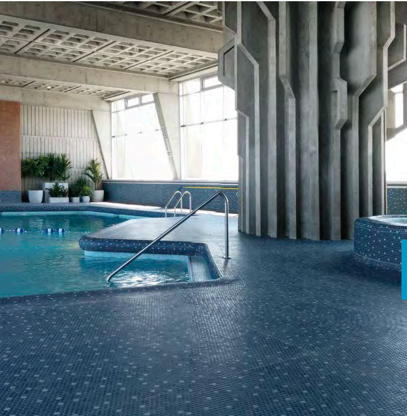
Indoor pool, Dauphins-sur-le-Parc, Montreal, Canada / Architects: Lapointe Magne & associés The pool is distinguished by almost 900 m 2 of Jasba-LOOP tiles. Loop (2 cm in diameter) was laid in Light Aqua Blue glossy and Secura in the pool. The architects selected a special Loop design in dark-blue with individual light-blue tiles for the pool surround as far as the ancillary areas.
